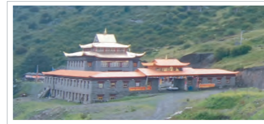
Kangding 392kWh Photovoltaic Off-grid Energy Storage Project
