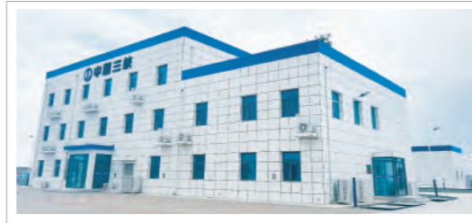
Ulanqab 180MWh Green Power Station Demonstration Project
