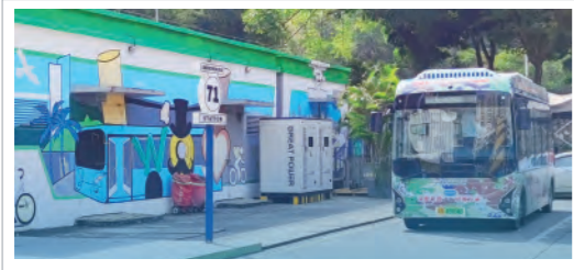
Croatia 17MWh Photovoltaic and Storage Complementary Project
