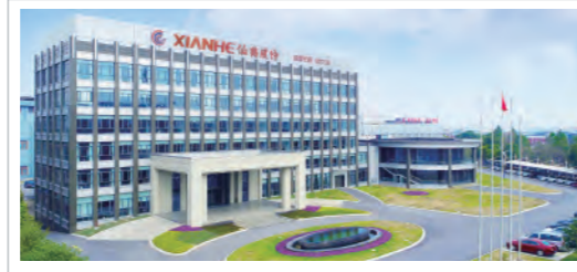
Zhejiang Xianhe New Energy Co., LTD. 44.72MWh Energy Storage Project
