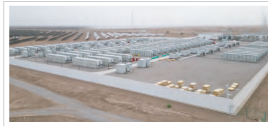
Bachu 140MWh Agro-Photovoltaic Complementary Project
